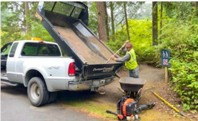
Raymond starting the upgrade work on our Kala Point forest trails.
