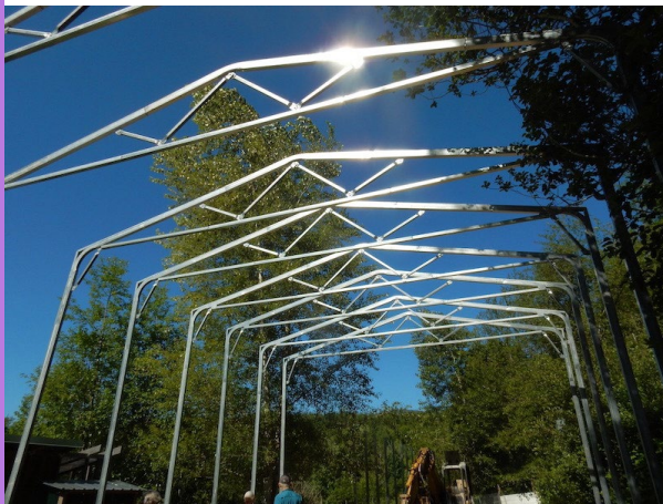
CVAR Aviary Structure: photo by Michael Hoskins
