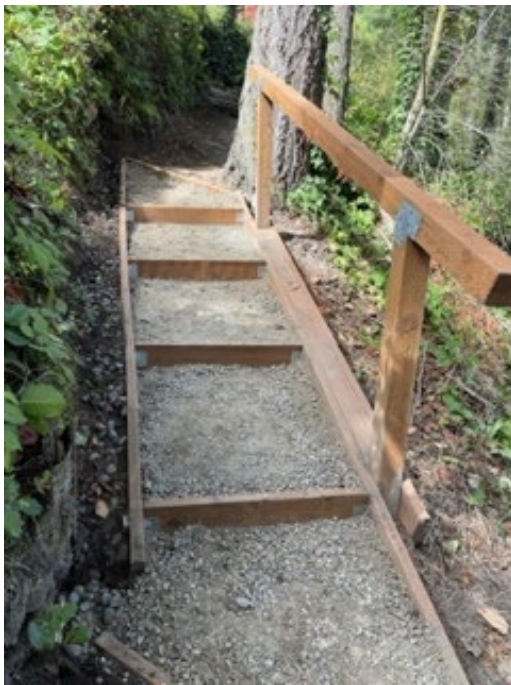
Newly repaired trail below Bluffs Drive
